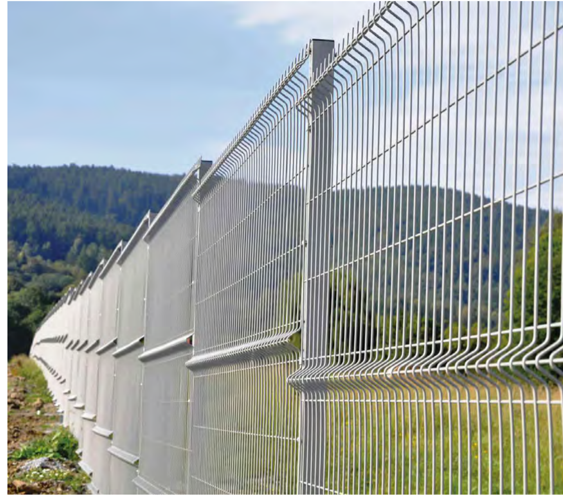
WELDED MESH FENCE EXAMPLE
